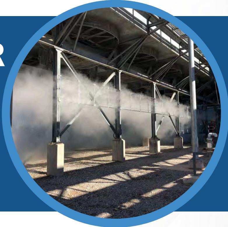
**MicroCool C3 systems improve heat rejection to help air cooled condensers maintain capacity under high ambient conditions.**
